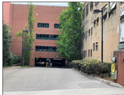
Walnut St (east) entrance of Locust Garage
