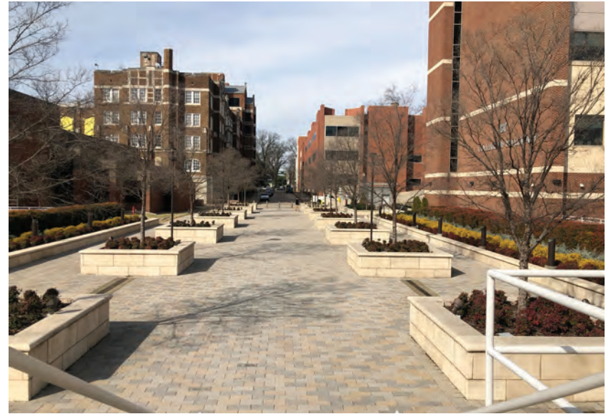
Pedestrian Extension at Monroe Avenue
